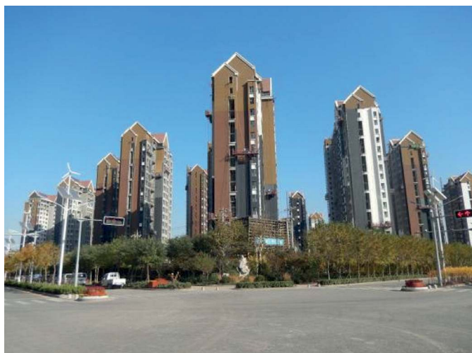
Photo 2 – The SSTEAC Southern Zone © R. Curien, November 2013.
